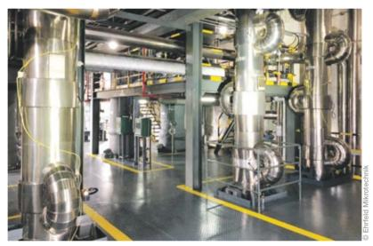
Integration of the continuously operating Miprowa flow reactors into the existing building infrastructure at Shaoxing Eastlake in China near Shanghai.
